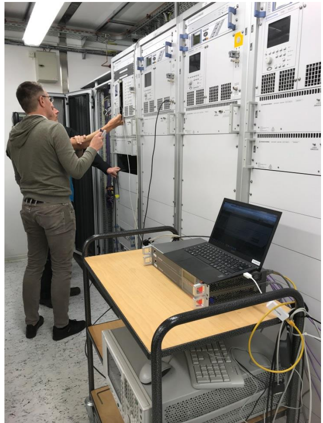
R&S 7000 upgrade – The Netherlands. N+1 TWISTER solution Improved MER from 39dB to 43dB!
