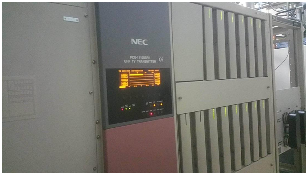
NEC analog PCU 1110SSP/A 800W Transmitter Upgrade with TWISTER from analog to Digital DVB-T/T2 – VietNam
