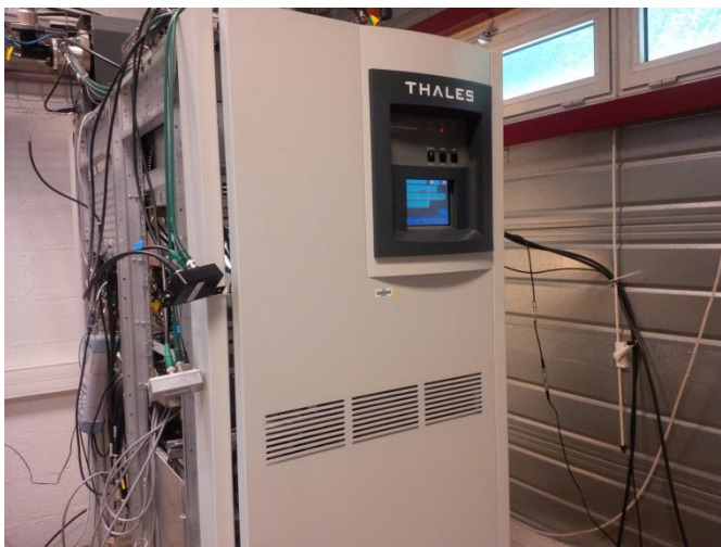
Thales 1200W DVB-T to DVBT/T2 upgrade - France. DualDrive TWISTER solution.
